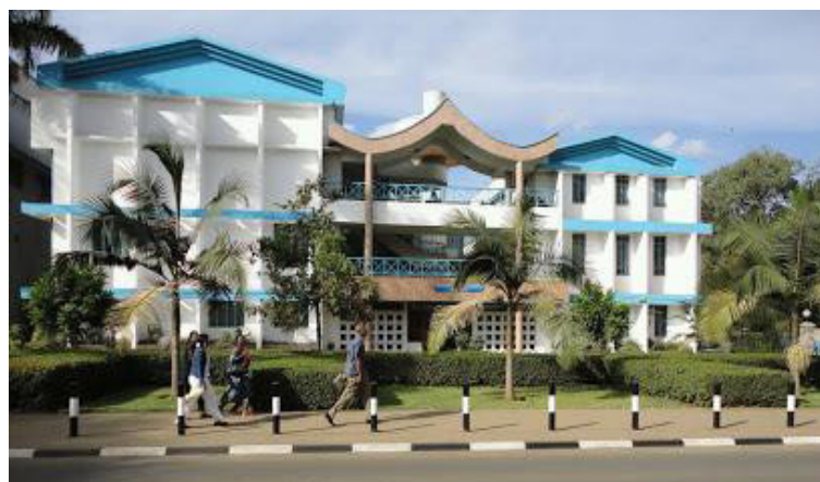
Figure 2.2: A picture of Civil Block.
