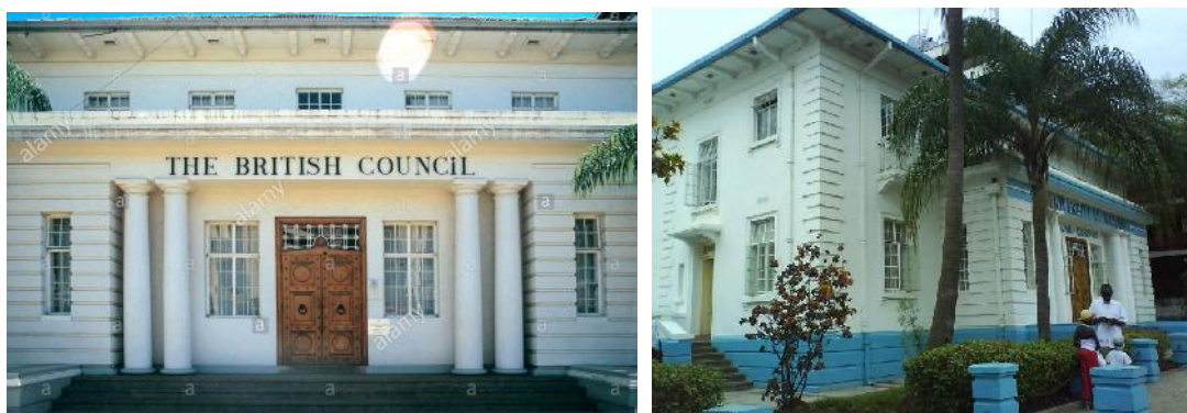
A views of the British Council Library Building in Kisumu which was transferred to the University of Nairobi in 2006
